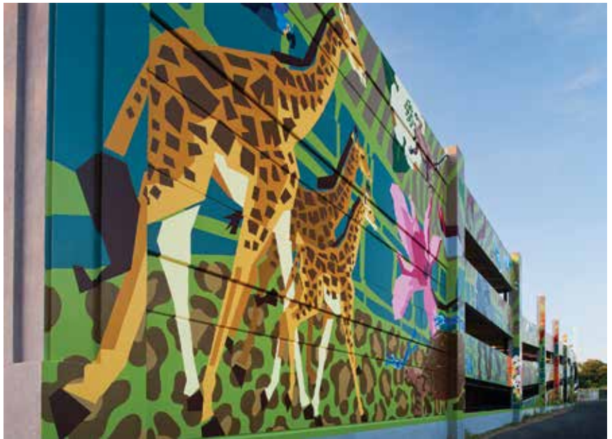
Large murals decorate the façade of the new precast concrete parking structure at the Philadelphia Zoo Centennial District Intermodal Facility. The project added parking while improving traffic flow and creating a community-centric plaza. Photo: Steve Wolfe Photography.
