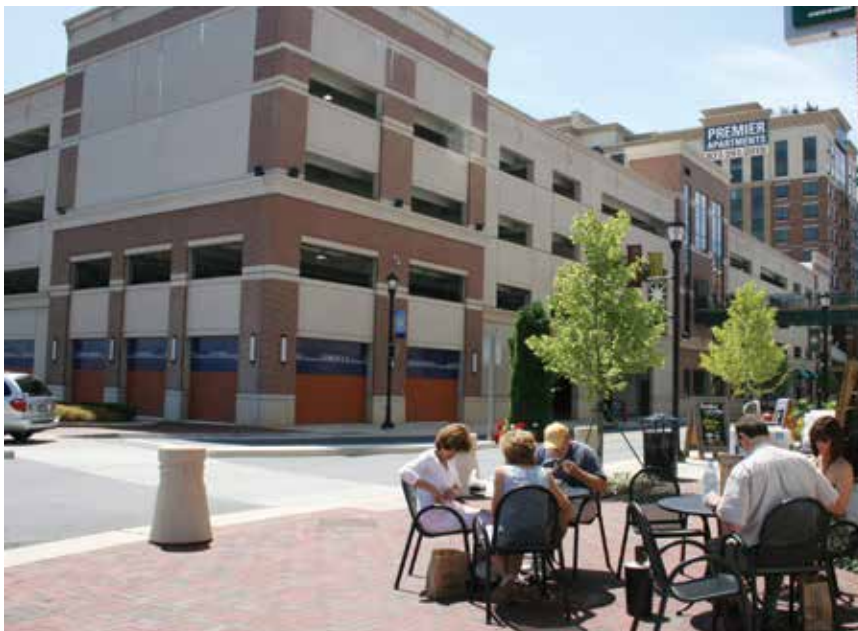
The Annapolis Towne Centre Garage provides dedicated spaces that help support the wide variety of uses for the facility, including banking, retail, condominiums, apartments, luxury hotel, fitness center, office space, and restaurants. Photo: TimHaahs.
